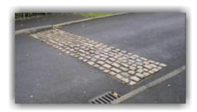
Rumble devices come in a variety of forms, which have been described as rumble strips, riblines, jiggle bars, rumble areas, RippleprintTM and rumblewave as well as cobbled or moulded road surfacing.
